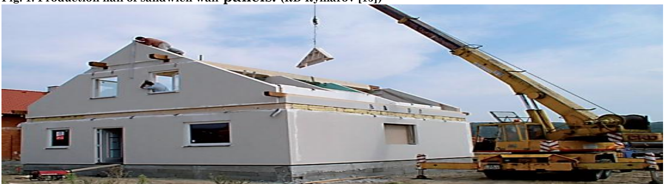
Fig. 2: Construction of panel construction system. (HAAS Fertigbau [16])
