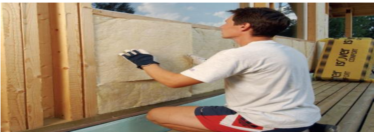
Fig. 4: Inserting thermal insulation of walls.
