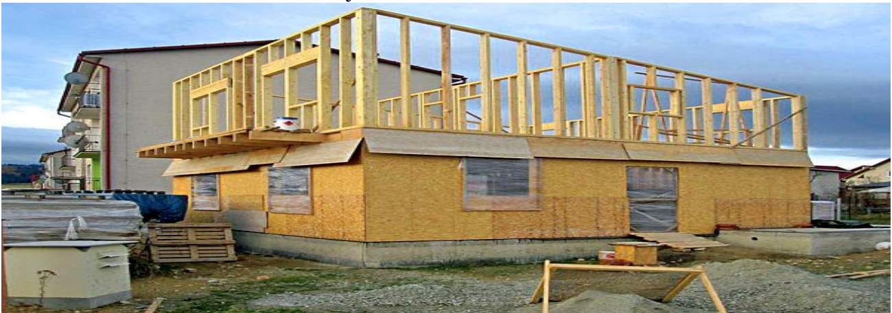
Fig. 3: Columnar construction system (Dubjel and Bobeková [17])
